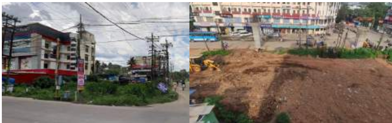
Figure 5-8: Existing site condition
