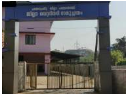
Figure 3-23: District Veterinary Hospital
