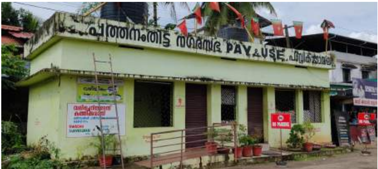
Figure 2-39: Existing Public Comfort station at old bus stand
