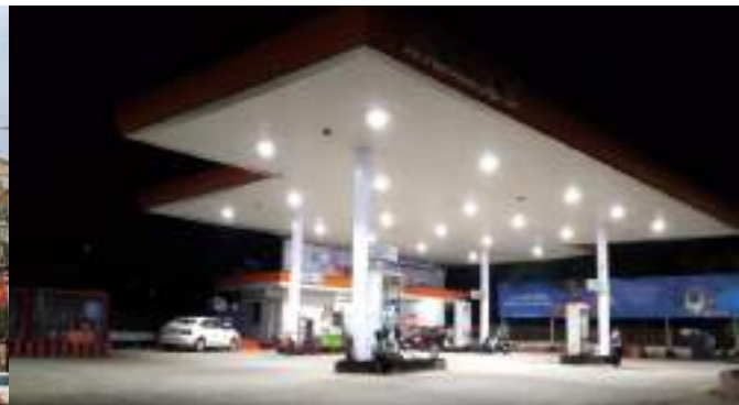
Figure 3-13: Fuel Filling Station
