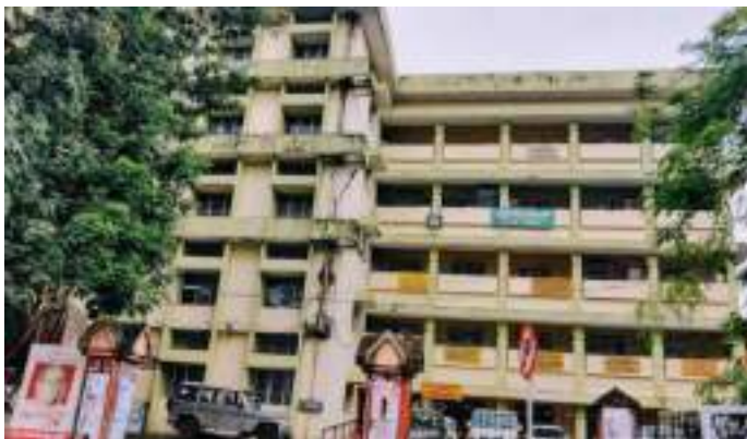
Figure 3-27: Mini Civil Station
