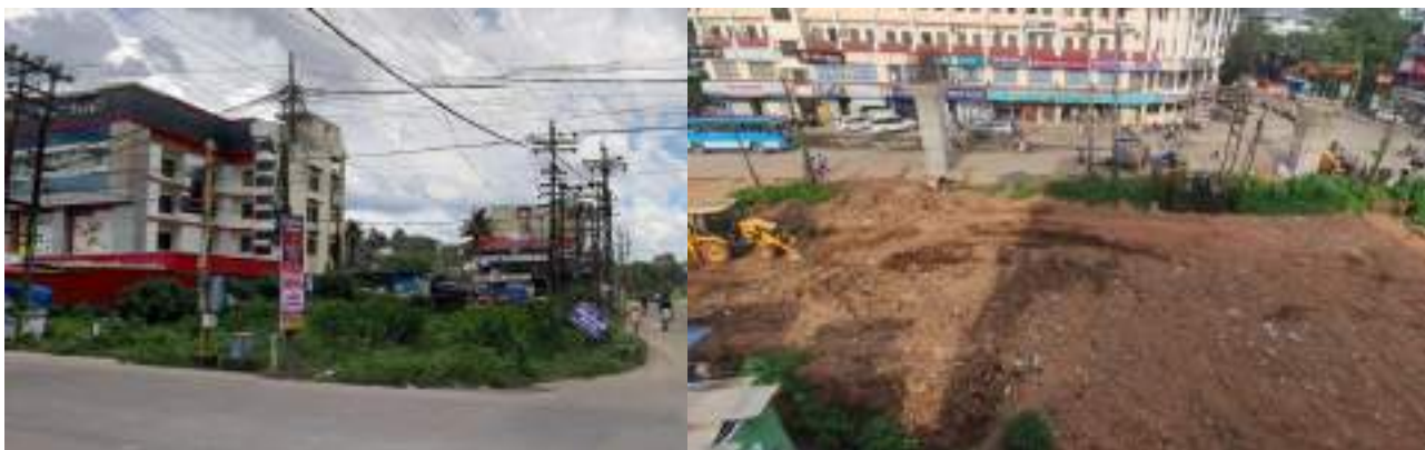
Figure 5-8: Existing site condition
