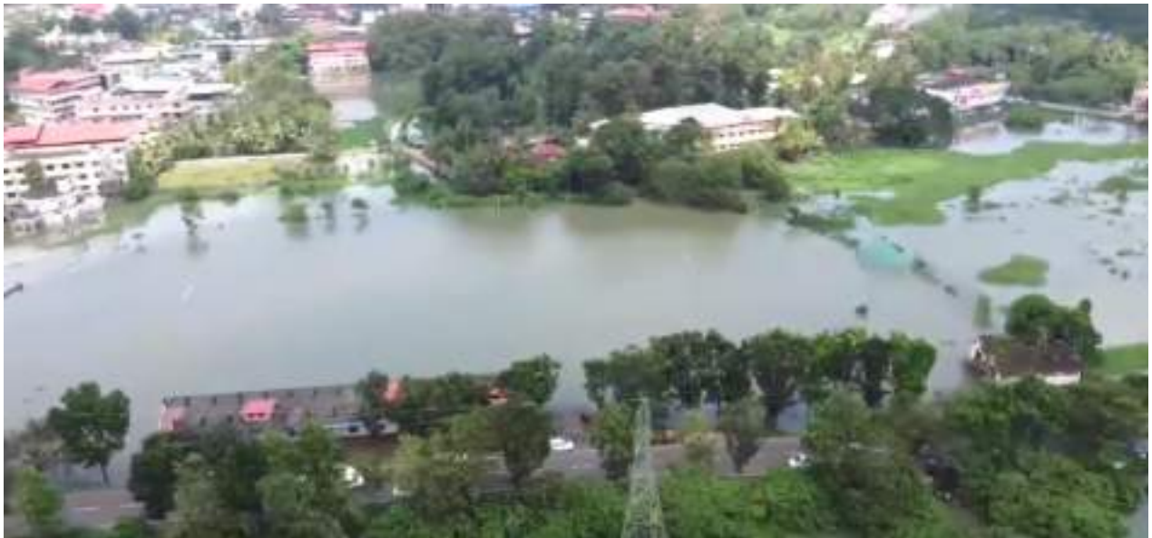
Figure 2-45: Flood in Pathanamthitta town
