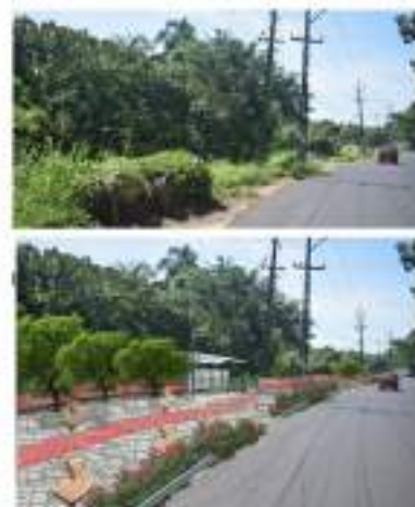
Before and after conditions of the Zone-4 Area
