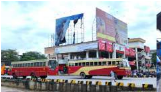
Figure 2-22: KSRTC Bus Terminal
