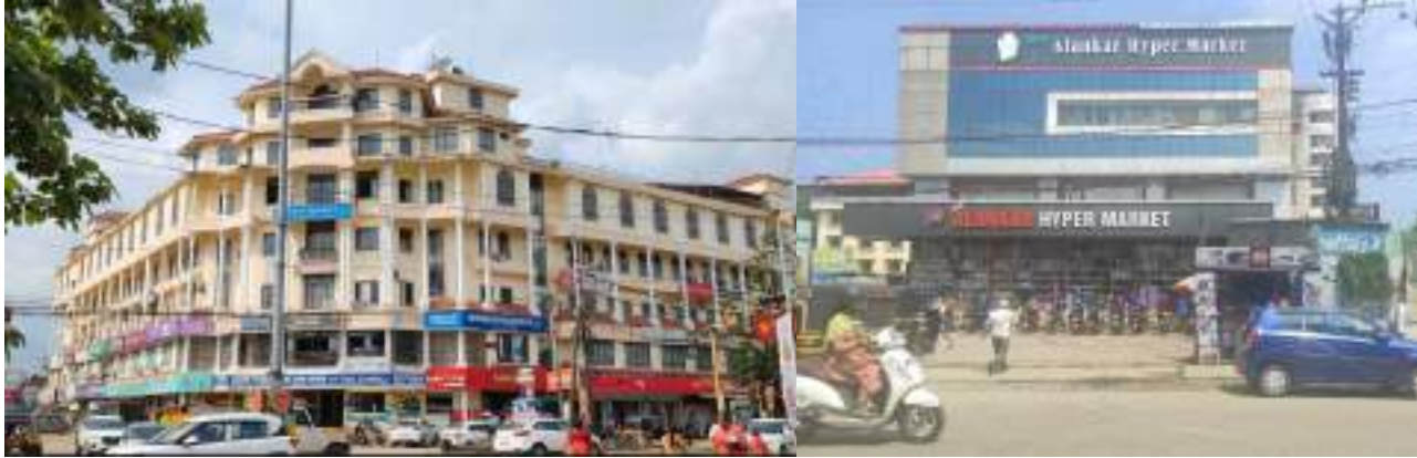
Figure 2-31: Major Commercial buildings in Planning area
