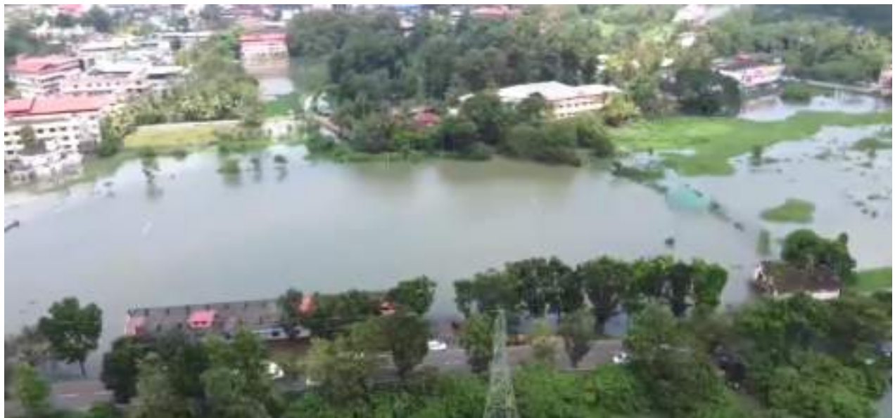
Figure 2-45: Flood in Pathanamthitta town
