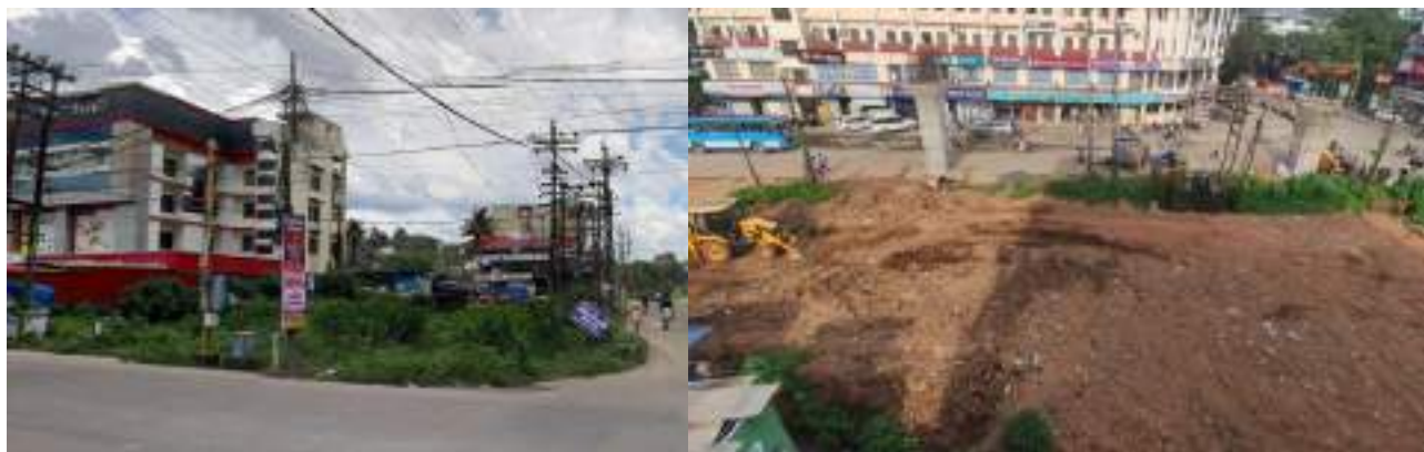
Figure 5-8: Existing site condition
