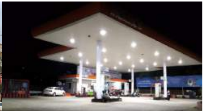
Figure 3-13: Fuel Filling Station
