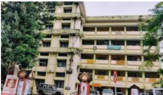
Figure 3-27: Mini Civil Station
