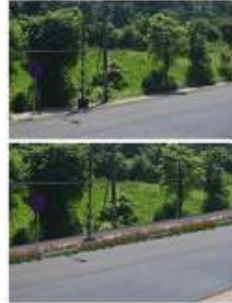
Before and after conditions of the Zone-2 Area
