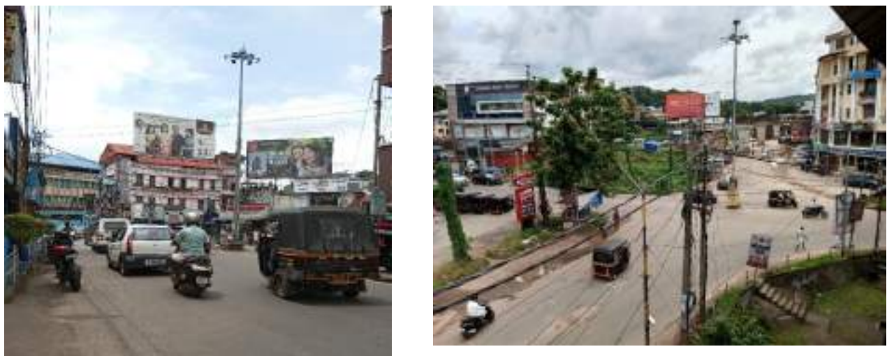
Figure 2-27: High Mast lights in junctions
