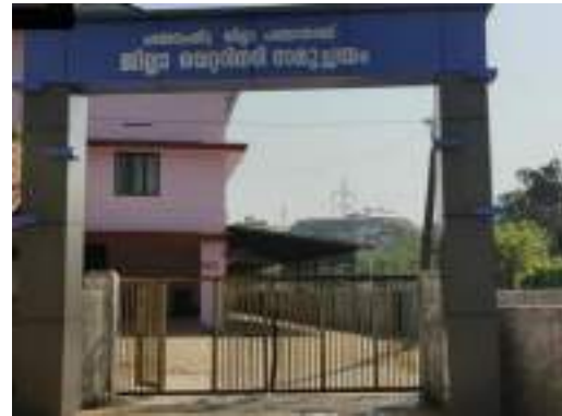
Figure 3-23: District Veterinary Hospital
