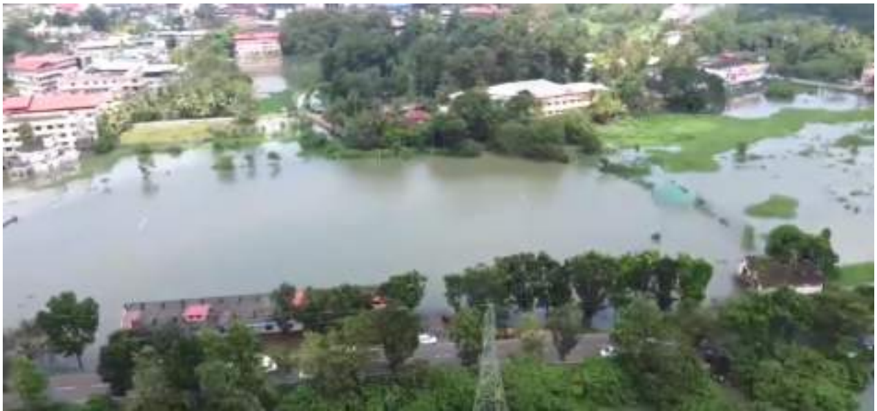
Figure 2-45: Flood in Pathanamthitta town
