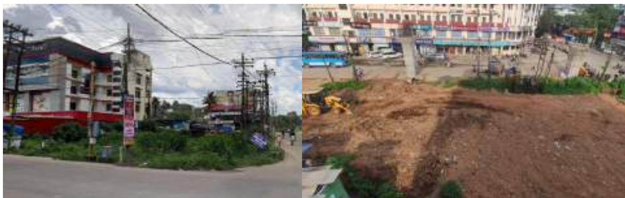
Figure 5-8: Existing site condition
