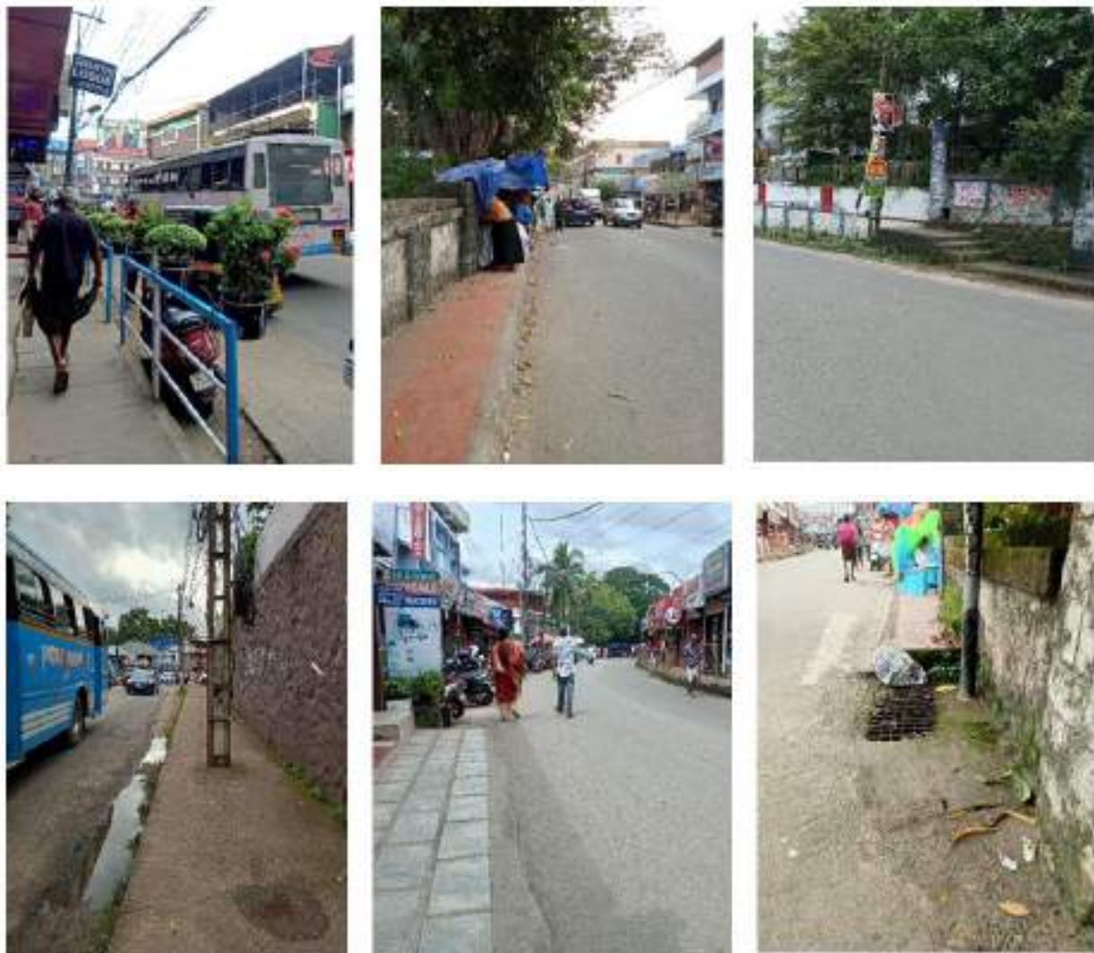
Figure 2-10: Existing Foot path condition in the Planning area
