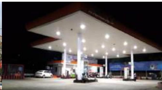
Figure 3-13: Fuel Filling Station
