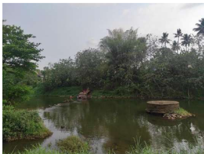
Figure 3.4: Intake for the water supply
