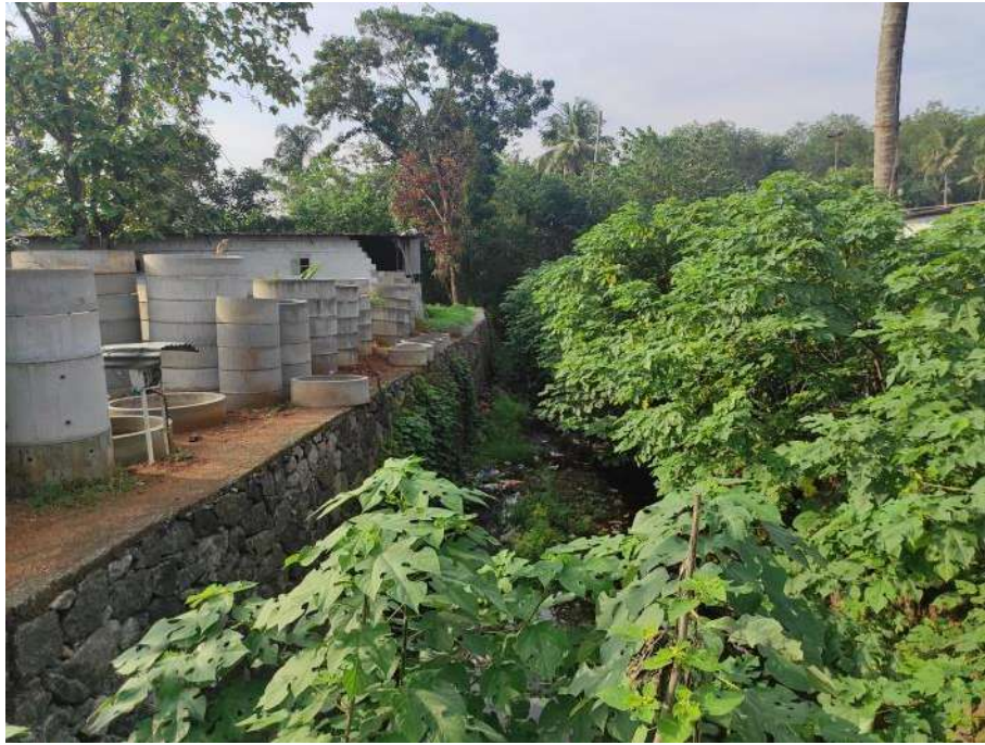
Figure 3.3: Natural drainage flows towards Achankovil River
